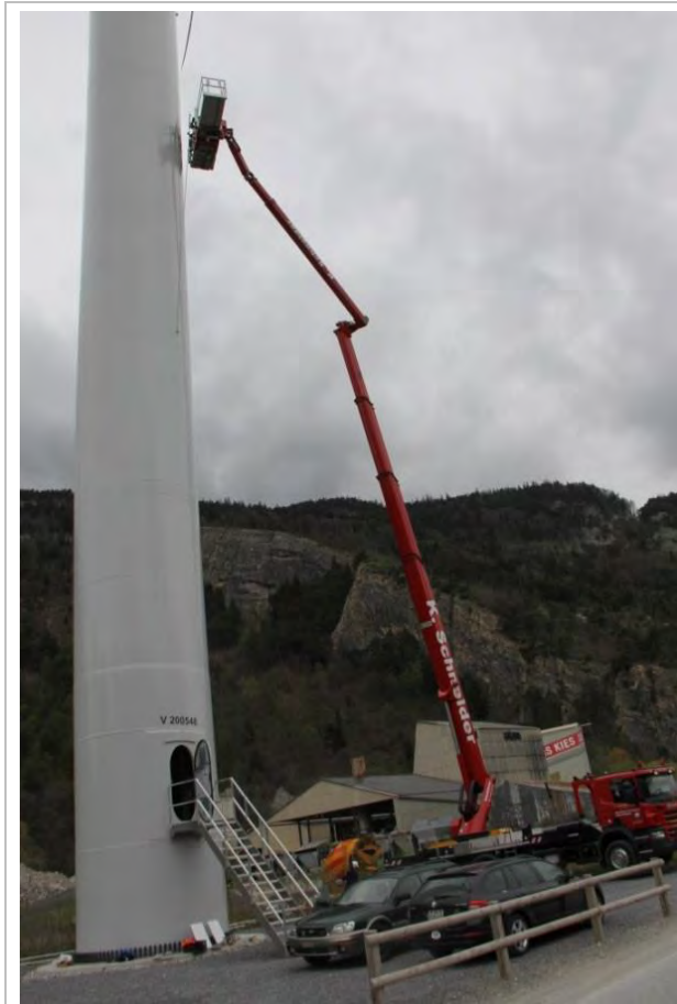
Installation at 31m height with man-lift
